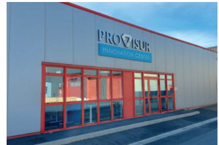
Development and testing can now be conducted at Provisur's newly opened Innovation Center (PIC) in Plailly near Paris
